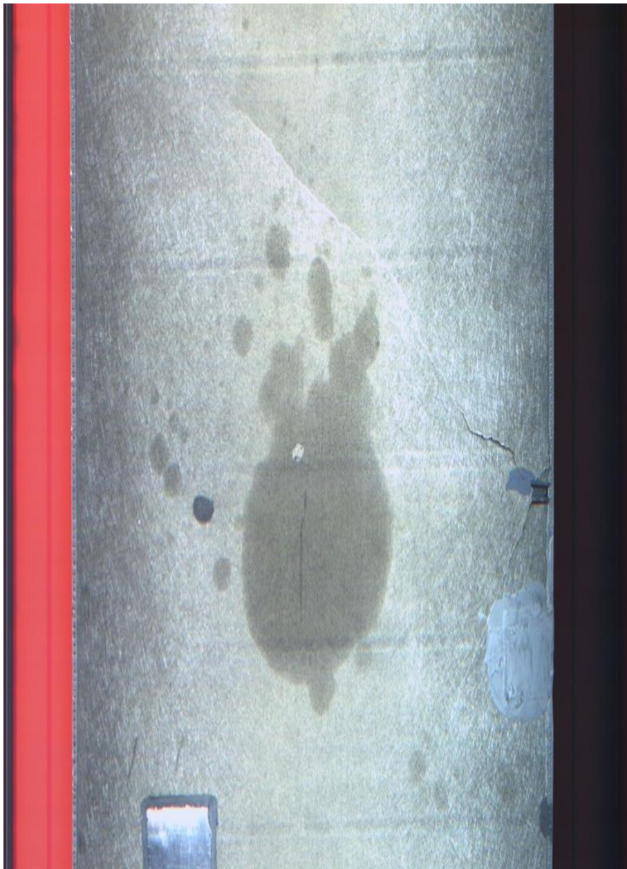
Roof Sheet Flex Crack – in gate
